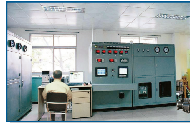
Performance Testing Centre
